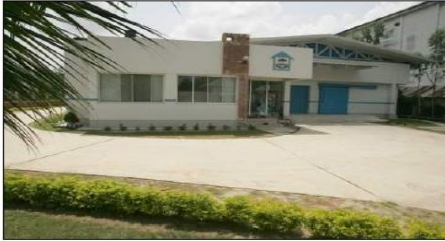
Grameen Danone Foods, Bogra Plant, Exterior
