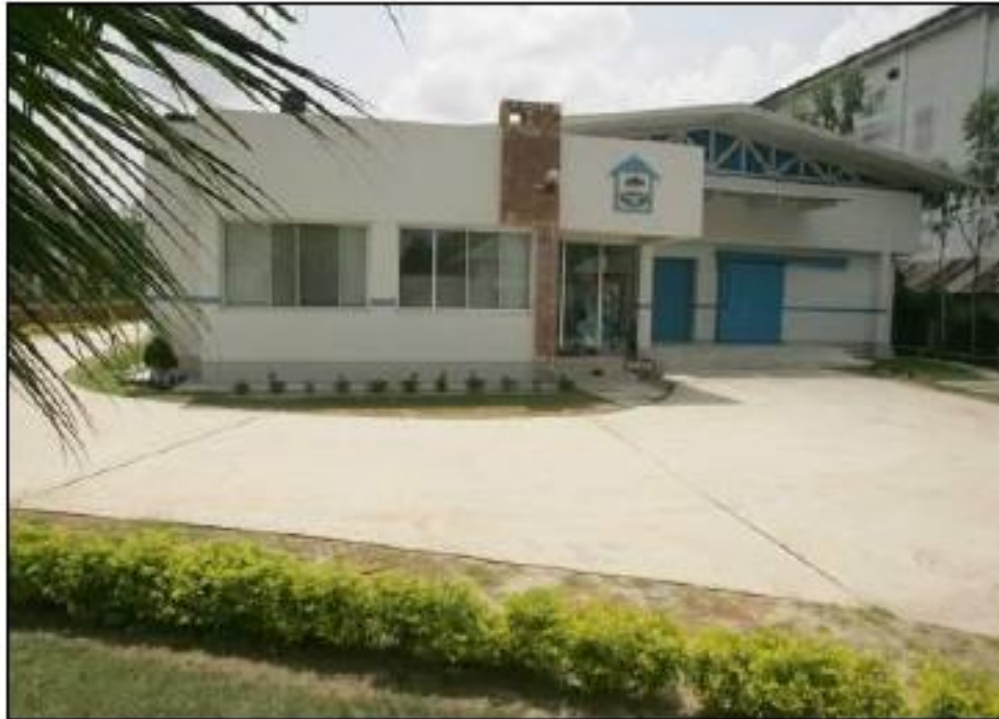
Grameen Danone Foods, Bogra Plant, Exterior
